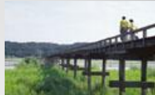
Horai Bridge (World's longest wooden Bridge:897m)
